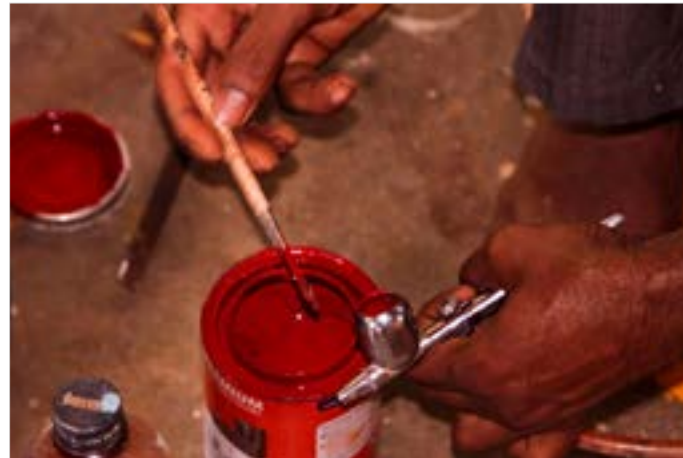
Turpentine is added to acquire the required viscosity of the paint.
