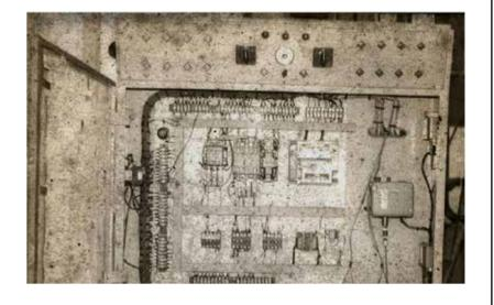
The control panel was thin in depth, lacked the visual weight as related to the Boiler! controls were not grouped functionally. They were distributed on either side of central line to make it symmetrical. The panel was sloping inwards, making it difficult see and operate. the chin down panel was not speaking out!
